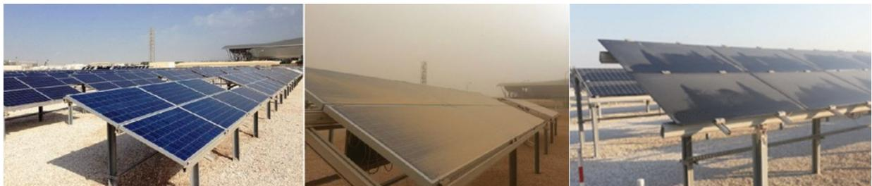
**Figure 1.5:** PV Panels in a solar power plant in Qatar [15]. Mud formation can be observed in the center and right photograph.
