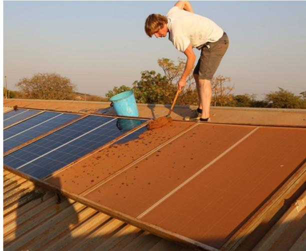
**Figure 1.8:** Dust adhesion on PV panels due to dew formation and exposure to dusty winds [42].
